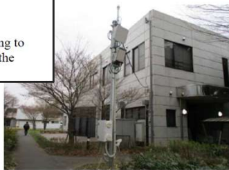
Figure 3.4 A base station facility constructed in the Tokyo-site
